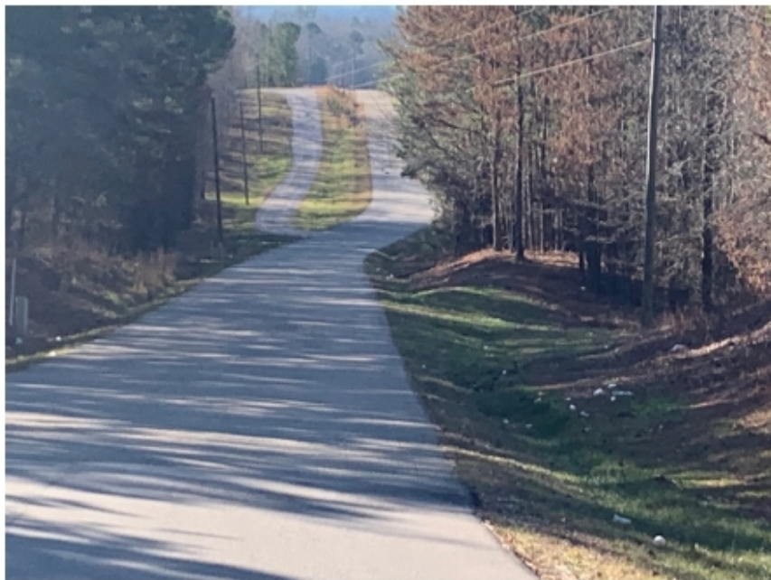
VIEW LOOKING SOUTH ALONG WHIPPOORWILL RD
