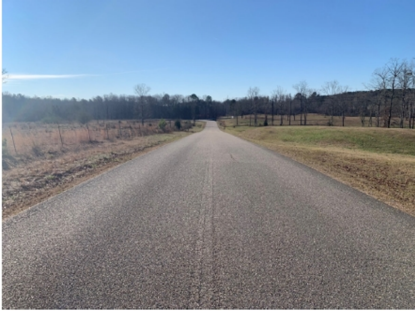
VIEW LOOKING SOUTH ALONG WHIPPOORWILL RD
