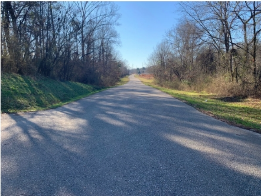
VIEW LOOKING SOUTH ALONG WHIPPOORWILL RD
