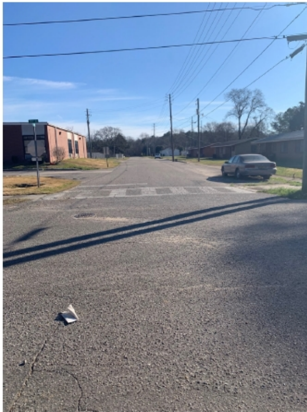
VIEW LOOKING NORTH AT SOUTHERN END
